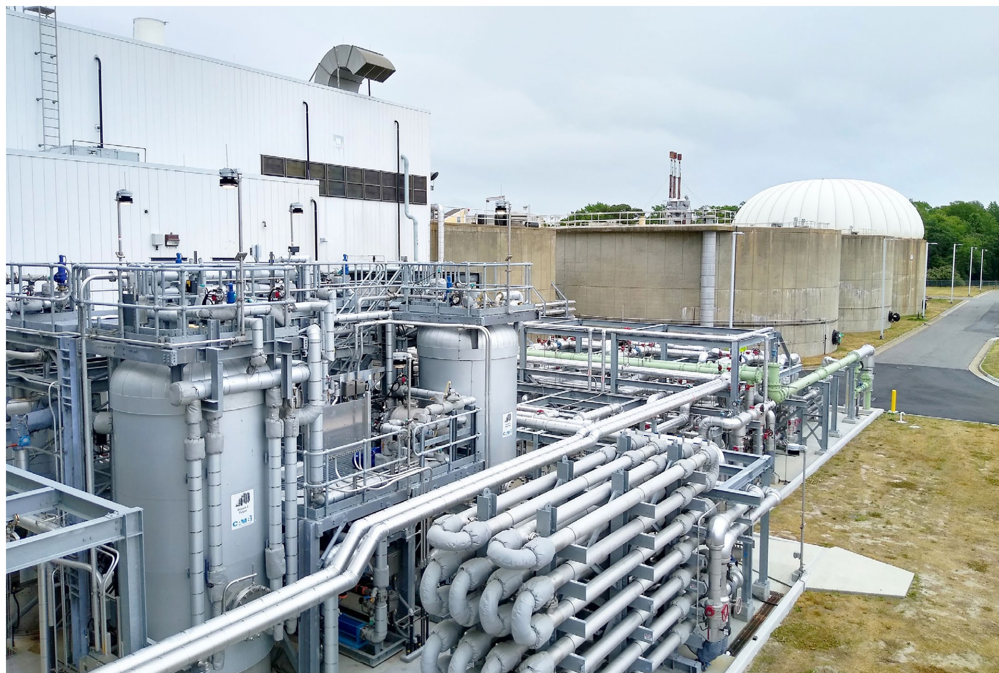
Thermal Hydrolysis Process System.
