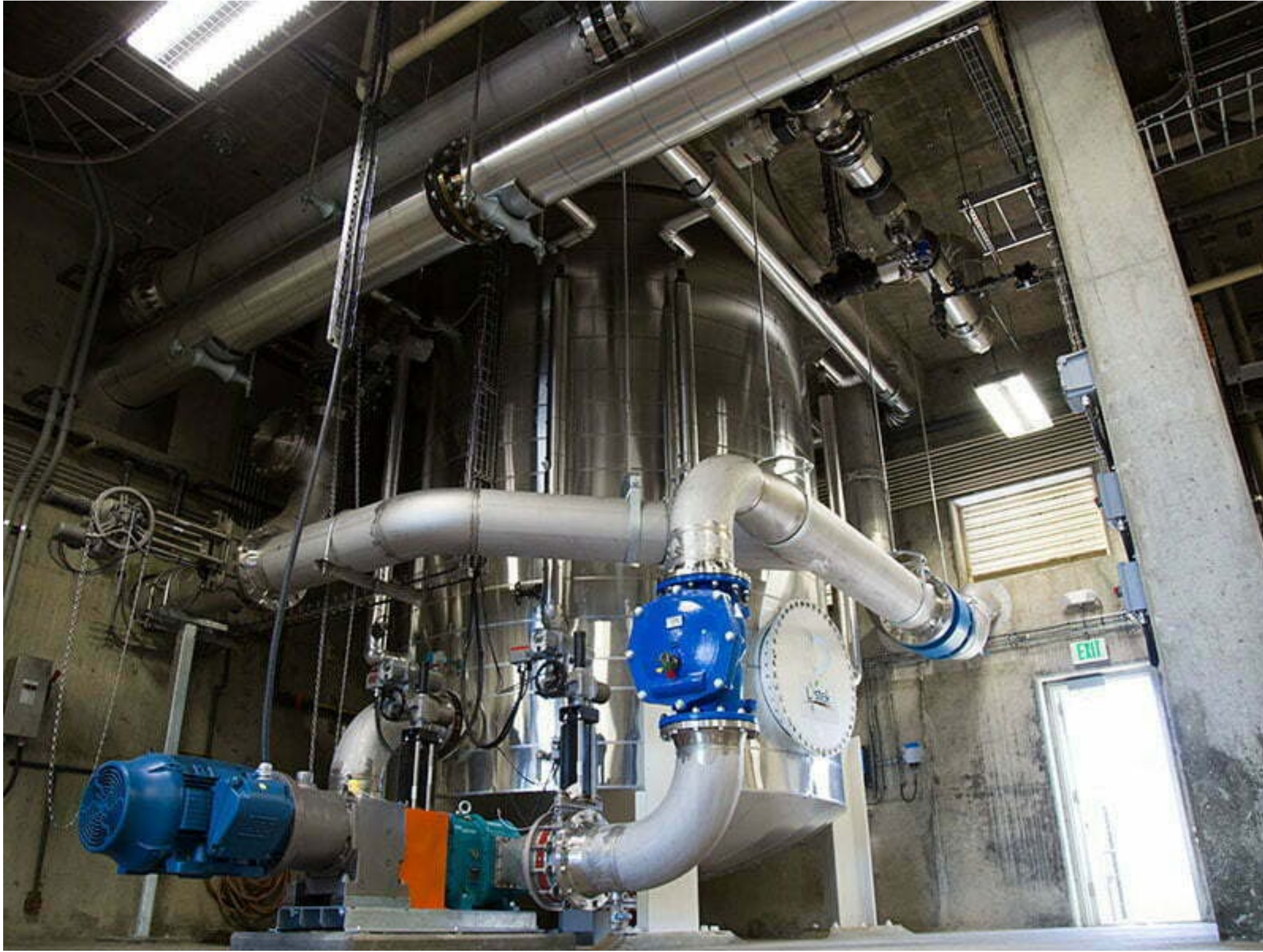
Thermochemical Hydrolysis System Reactor.
