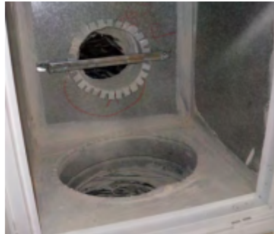
Well-sealed return with mastic fully covering seams, duct connection, and interior of duct
