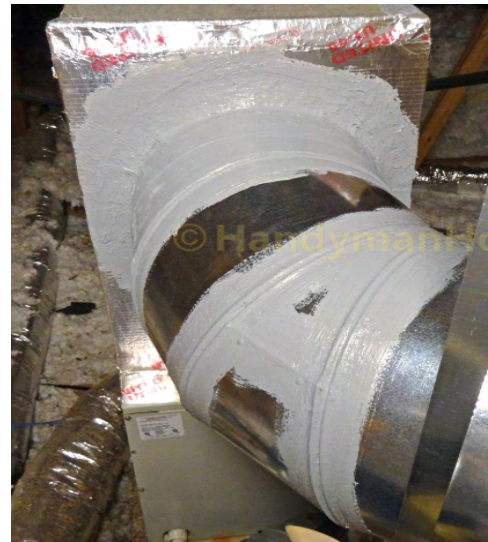
Well-sealed metal duct - all connections and seams are sealed. Insulation has not yet been installed.
