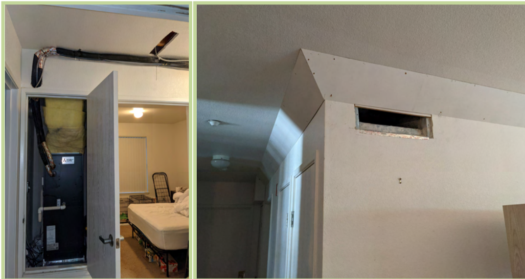
Figure 22: In progress view showing surface mount line set and hole in drywall to run new electrical (left); In progress photo showing line set hidden under cove trim in two-bedroom apartment (right)
