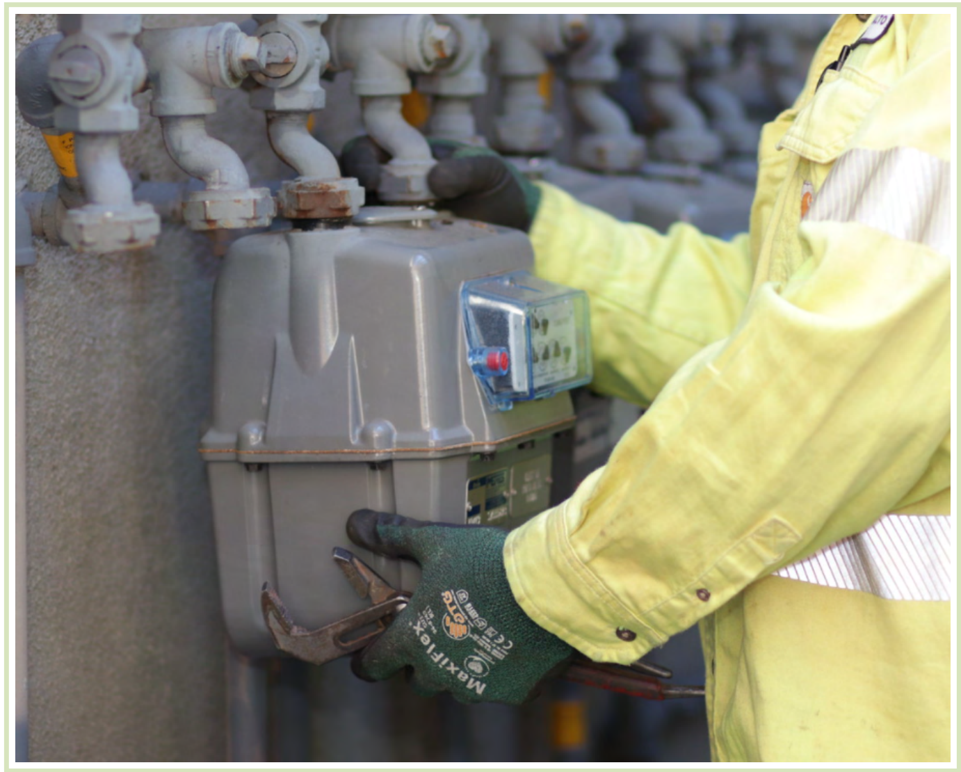
Figure 29: Removal of gas meter at project site
