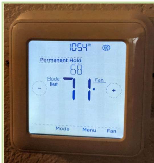
Figure 24: Thermostat used for both ducted and ductless heat pump installs
