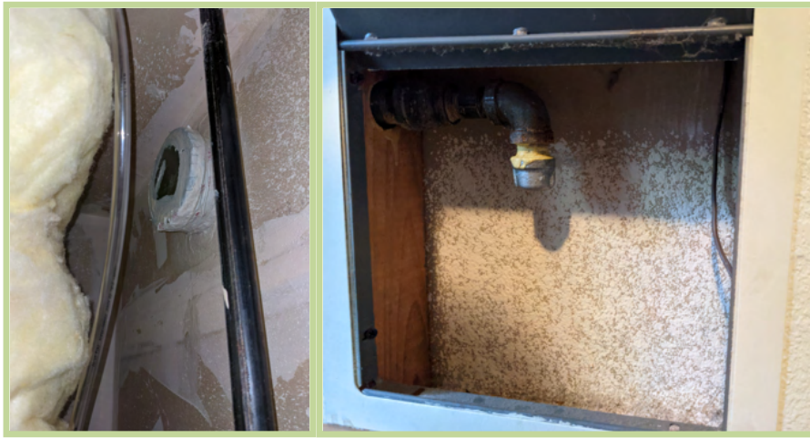
Figure 21: All combustion air openings and flue pathways were sealed in furnace closets as part of the retrofit (left); Typical gas line capping – all gas shut offs for wall furnace were accessible through access panels located in the bedroom (right)
