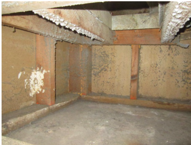
Plenum is unlined and unsealed
