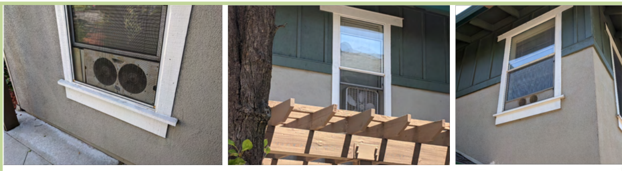
Figure 6: Fans and room AC units seen throughout the site to provide comfort cooling
