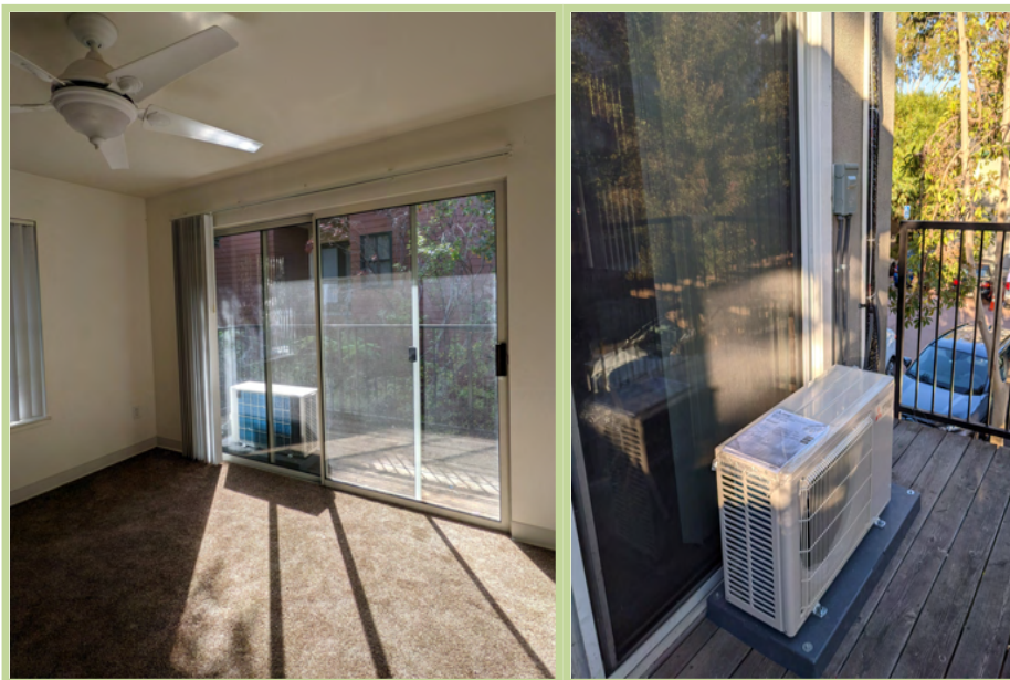
Figure 20: Typical one bedroom apartment showing compressor on deck in front of fixed sliding door pane
