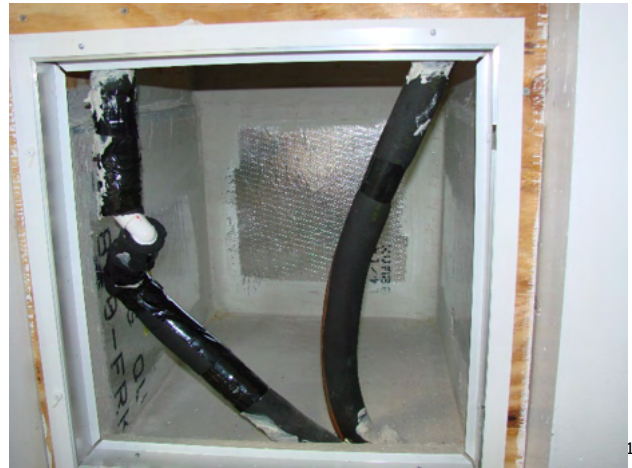
Plenum lined duct board and thoroughly sealed with duct mastic
