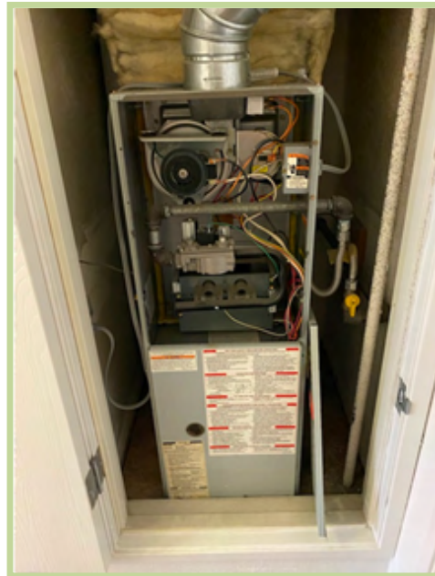
Figure 5: Typical gas forced furnace seen in two-bedroom apartments
