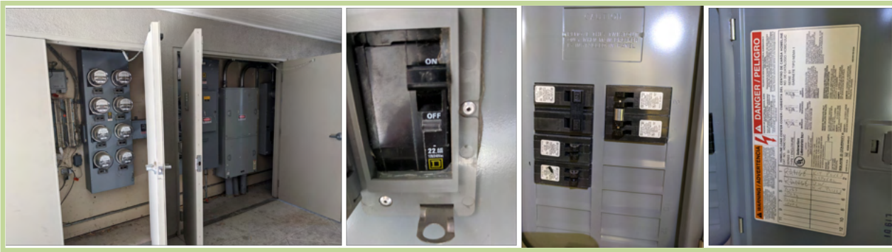
Figure 7: Existing electrical room (left), 70-amp apartment main breaker (center), typical apartment sub panel (right)
