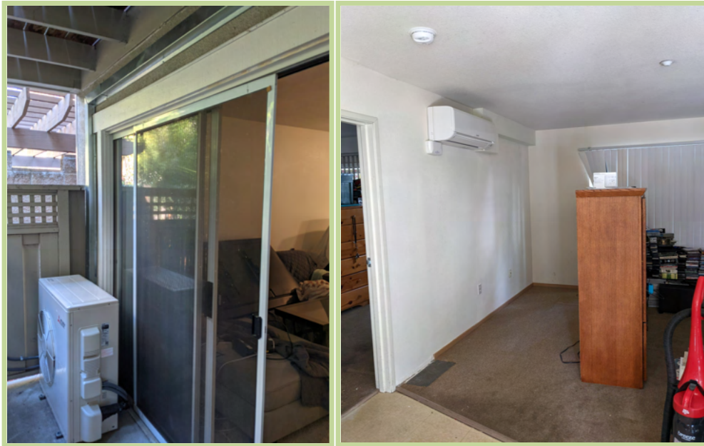
Figure 23: Typical (larger) two-bedroom compressor on patio (left); One bedroom unit with installed ductless fan coil, wall patched, line set cover boxed out (right)
