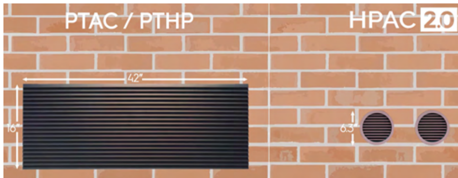
Figure 19: Image Courtesy of Ephoca Website, two holes shown on right represent Ephoca termination, image on left represents a typical package terminal heat pump termination
