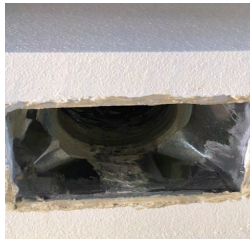
Supply boot and duct connection are well sealed with mastic; boot sealed to drywall with mastic or caulking
