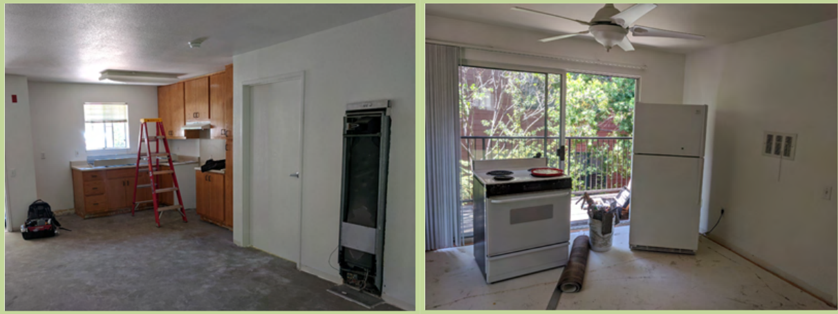
Figure 4: Typical one bedroom apartment showing wall furnace (covered removed) in living room (left), and rear vent in bedroom (right)
