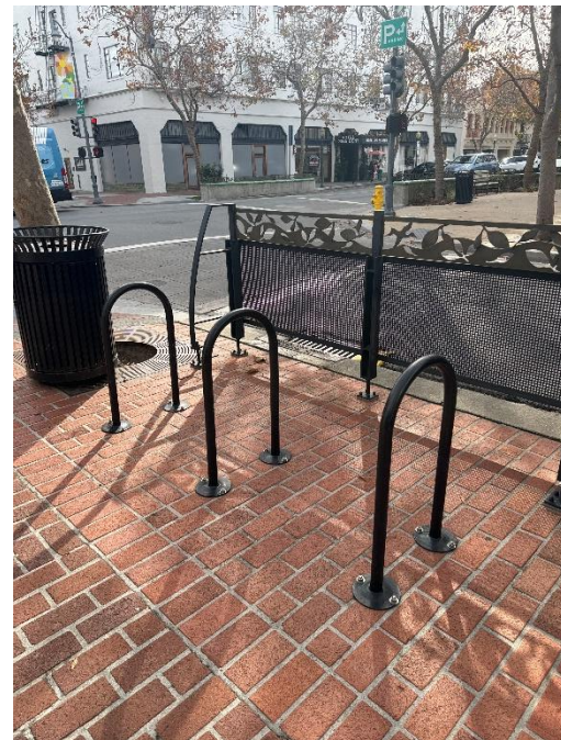
B. Not Secured to Ground
