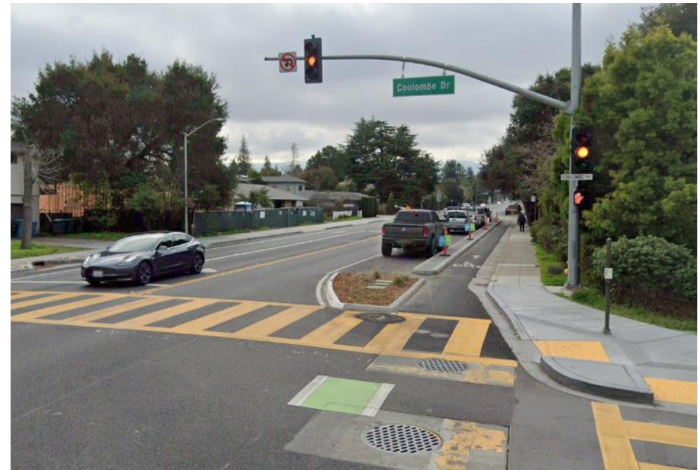
Photo: Arastradero Road south of Coulombe Drive Foto: Arastradero Road sur de Coulombe Drive
