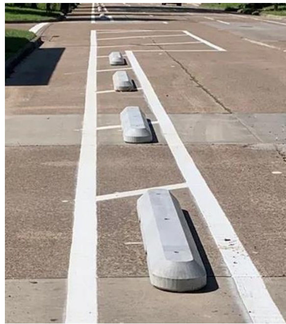
Photo: Concrete curbs
