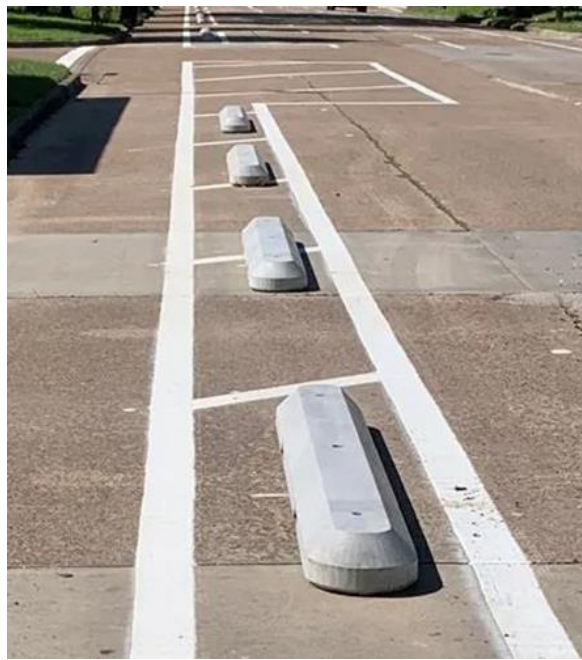
Photo: Concrete curbs
