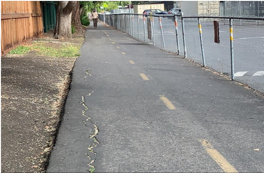
Photo: View of existing path and fence Foto: Vista del sendero y valla existentes
