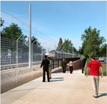
1 Example 12' Wide Ramp at 7% Grade Parallel to Caltrain Tracks
