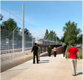
Example 12' Wide Ramp at 7% Grade Parallel to Caltrain Tracks
