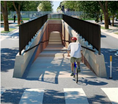
1 Example 12' Wide Ramp at 7% Grade Perpendicular to Caltrain Tracks
