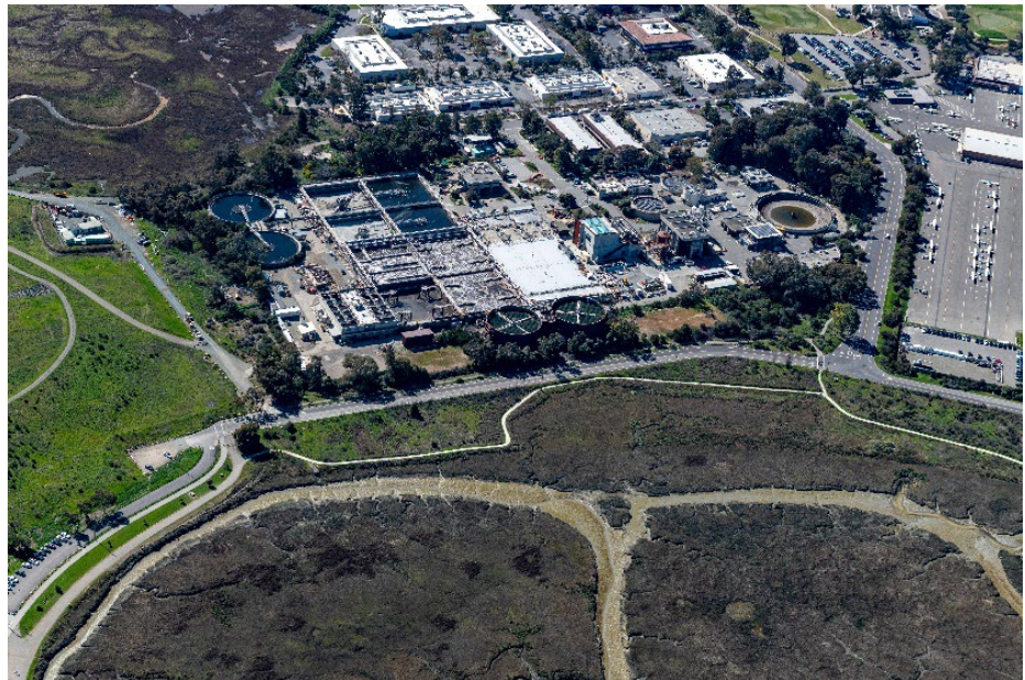
Aerial of the Palo Alto Regional Water Quality Control Plant and adjacent project area.
