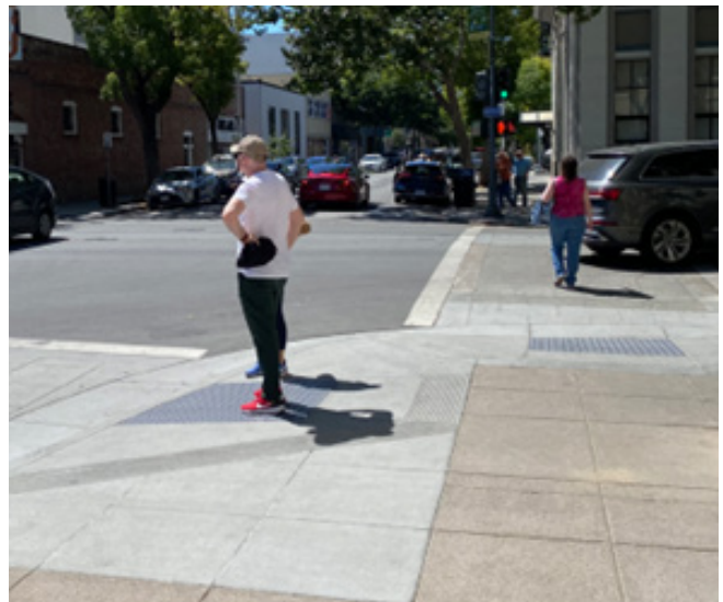
Marked crosswalks and curb ramps at University Avenue and Ramona Street.
